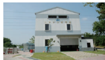
Hatta Power Plant
