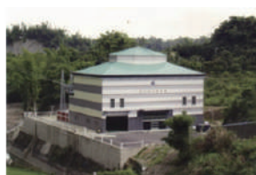
Xikou Power Plant
