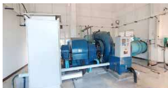
Installation of hydropower generator at Shalu Water Distribution Center
