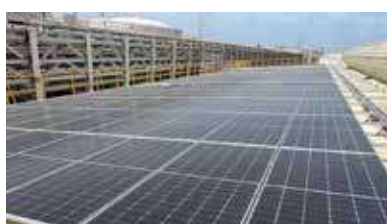
Installation of solar panels on the south rooftop of the acetic acid maintenance plant
