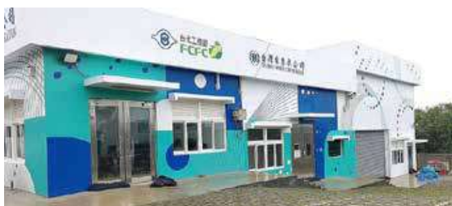
Installation of hydropower equipment at Shalu Water Distribution Center (plant building)
