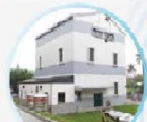
Batian Hydropower Plant 2,196 kW [2016]
